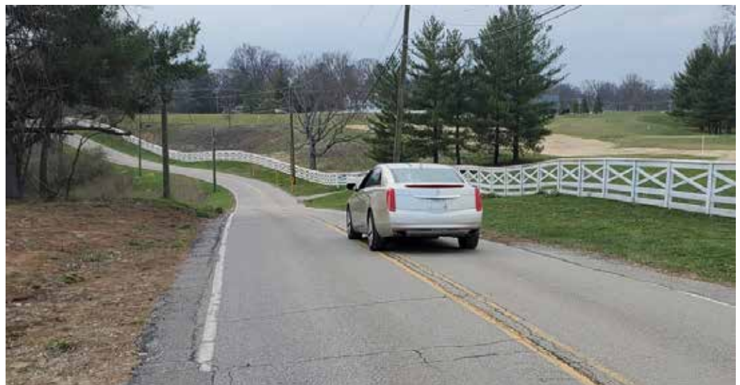
Ayers Road improvements
